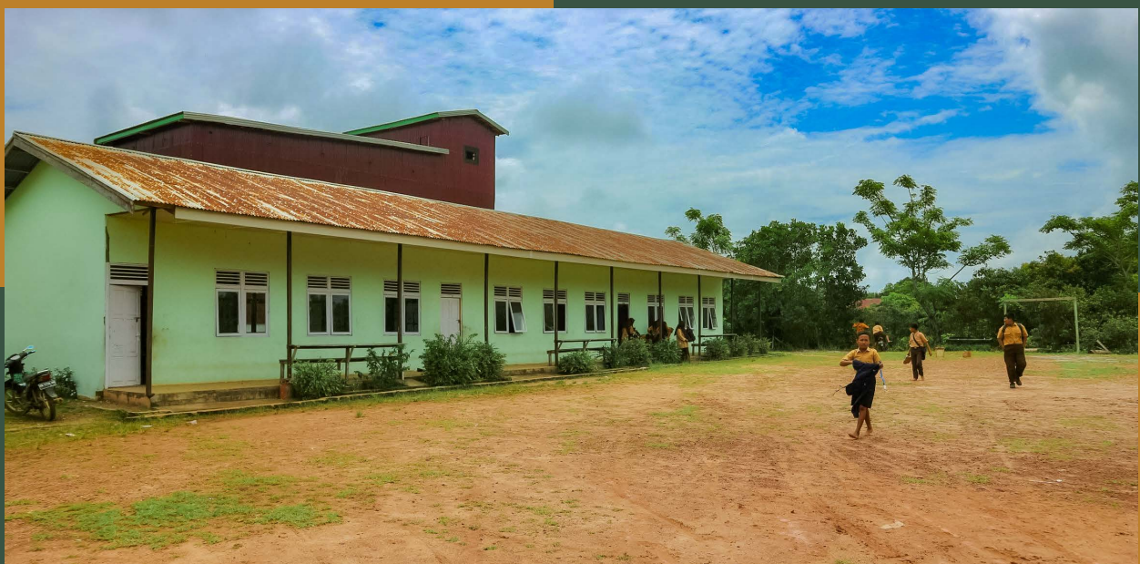
Additional classrooms at SDN 16 Kendawangan from Bumitama Berdaya Pendidikan
